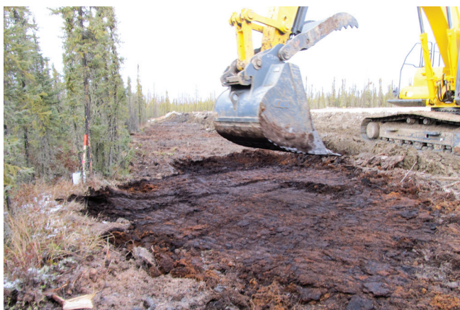
C. Inverted peat over buried clay being tapped and smoothed for a uniform surface. Note the smooth transition between the surrounding peatland and the recalimed surface.
