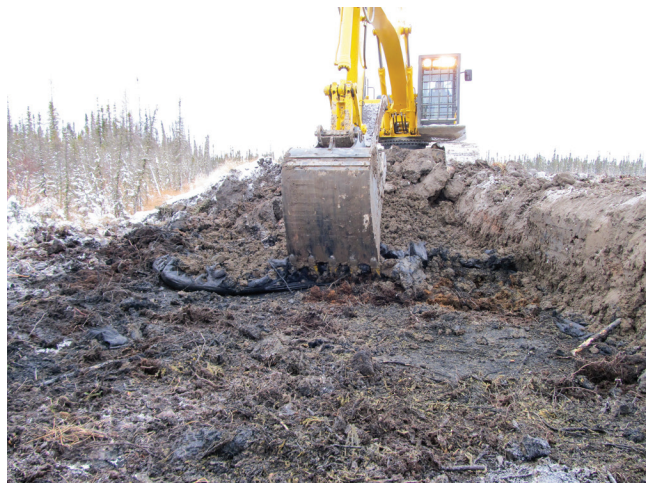
Figure 2. Clay pad material on the right waiting for removal. In the foreground, exposed peat as the geotextile is being peeled back by the hoe. Note the elevation differences between the surface of the clay (right), the exposed peat (middle) and the natural vegetation (left).
