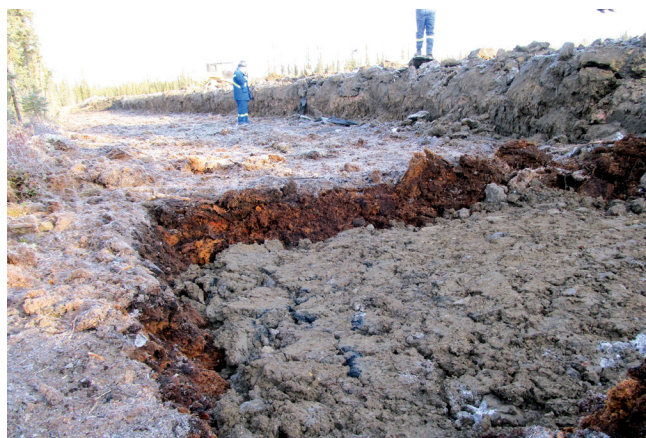
B. Clay has been replaced in the hole where peat had been excavated and placed on top.
