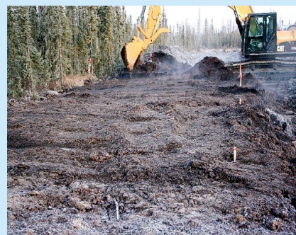
Figure 3. Left: The peat surface after clay removal waiting for fluffing. Right: The peat surface following fluffing.
