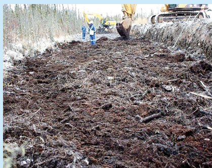
Figure 3. Left: The peat surface after clay removal waiting for fluffing. Right: The peat surface following fluffing.
