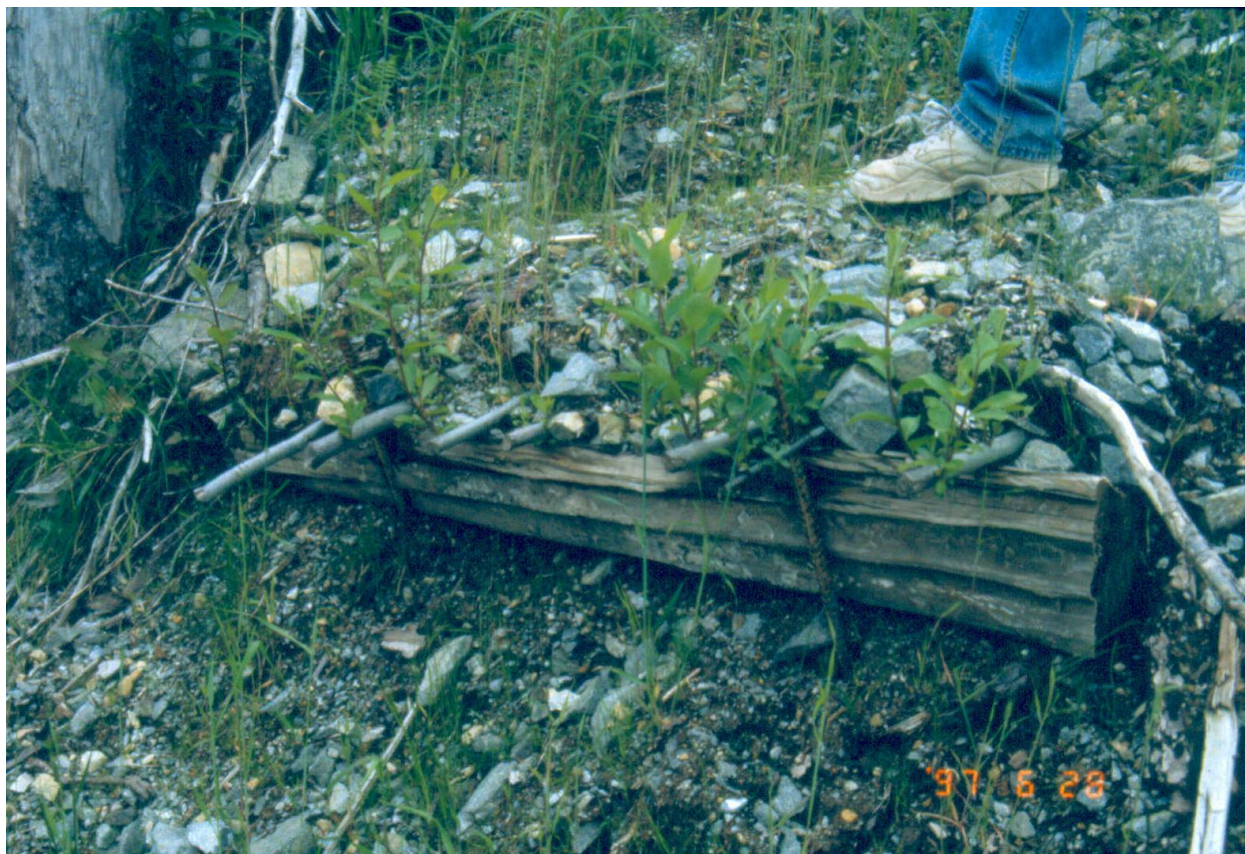
Photograph 4. Live pole drains can be used to treat moisture-related slumping sites.
