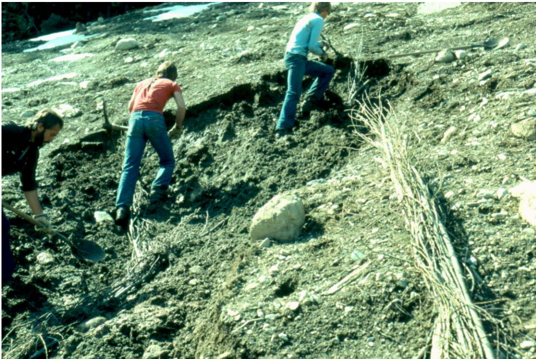
Photograph 3. Live pole drains can be used to treat moisture-related slumping sites.
