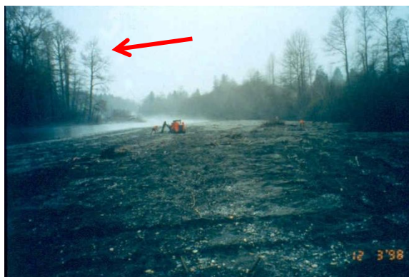
Figure 4. Live gravel bar staking is used to initiate natural succession on bare gravel bars. The sprouted cuttings trap small woody debris that in turn creates a flow disruption that results in deposition of sediment. Once the sediment builds to the point where the sprouts can no longer trap small woody debris there is no more sediment capture until the next year when growth of the sprout again traps woody debris.
