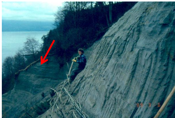
Photographs 1 (left) and 2 (right). Wattle fences were used to treat the sand cliffs at the University of British Columbia. Red arrows show an untreated buttress in the background.
