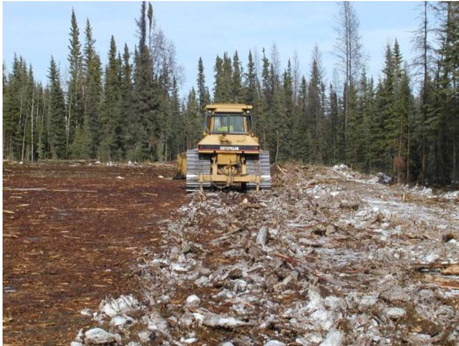
Figure 1. Straight shank ripping results in an effect similar to agricultural cultivation.
