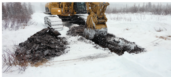
Wood chip burial: wood chip layer removed to side, with underlying peat being excavated to create a hole to bury the wood chips in.
