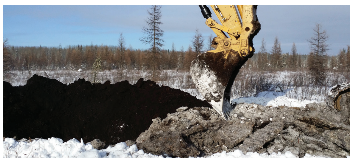
Wood chip burial: wood chip layer piled on right, with underlying peat substrate piled on left. Once the wood chips are placed in the hole, the excavated peat will be placed on top.
