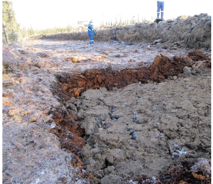
Clay pad removed, and mineral fill backfilled into excavated hole in the underlying peat, awaiting final replacement of peat on top.
