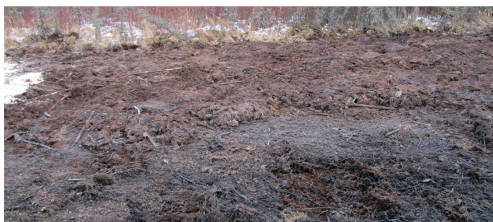
Clay burial: final peat surface at a similar elevation to the low points in the natural areas, awaiting revegetation.
