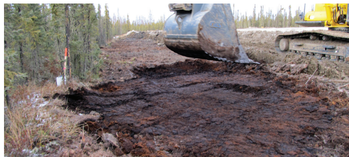
Clay burial: clay fill, completely buried under 40cm of peat substrate.
