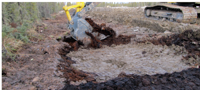
Clay burial: backfilled clay fill being buried under excavated peat to create final peat surface.
