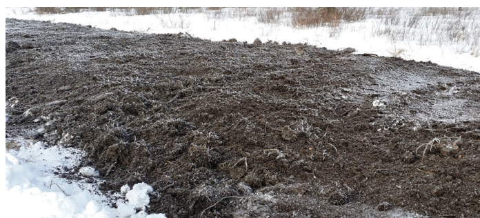
Wood chip burial: final peat surface after wood chip burial, awaiting elevation adjustment by trackpacking. Final surface elevation must be similar to that of the adjacent natural area to ensure proper moisture.
