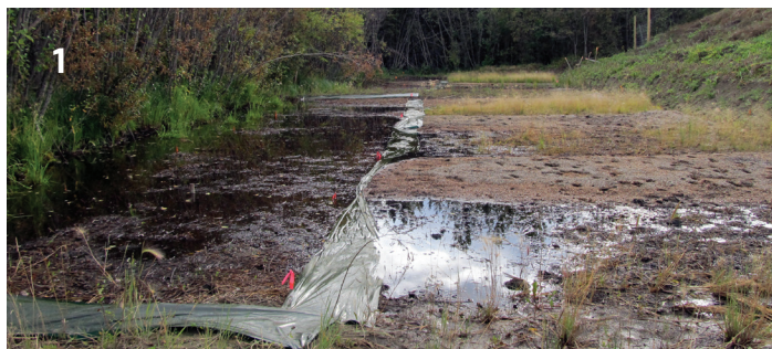
Completed soil preparation following partial pad removal (remaining pad on right) down to similar elevation as the peatland on left.
