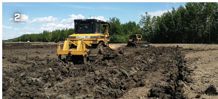
June 2014. Dozer with 1 m ripper shanks created microtopography with trenches to connect water flow across the site.
