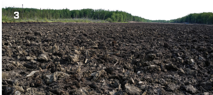
June 2014. Completed site surface prior to winter freeze thaw action. Amplitude was 150 cm from the highest points to lowest in the trenches.
