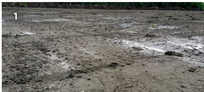
June 2014. Site surface lowered to desired elevation. Target elevation was 10 cm lower than the hollows/low points in a remaining wetland adjacent to the site.
