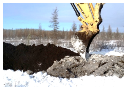
Figure 3. Stripping chips and piling of peat using a backhoe.
