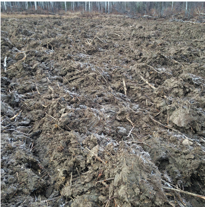
Figure 2. Site post-earthworks with soil stripping placement.
